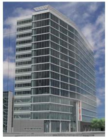
frames, located mainly in the rear of the building, resist lateral loads transferred by the rigid diaphragm. The most structurally challenging feature of Gateway Plaza is its 52'x36' bays. Preserving this open layout of the office is a major concern for the architect.
